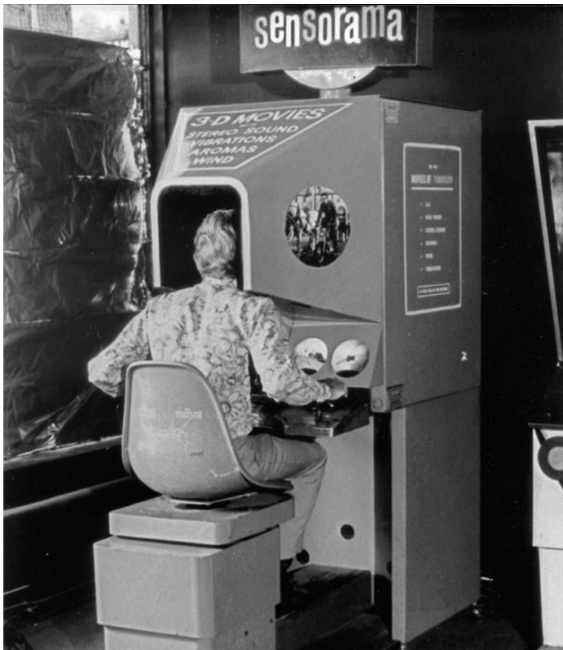
Figure 2.1: The sensorama allowed users to experience simulated senses. Users could experience stereo sound, vibrations, aromas, and wind. They would sit in a seat and immerse themselves within the device. [8]
