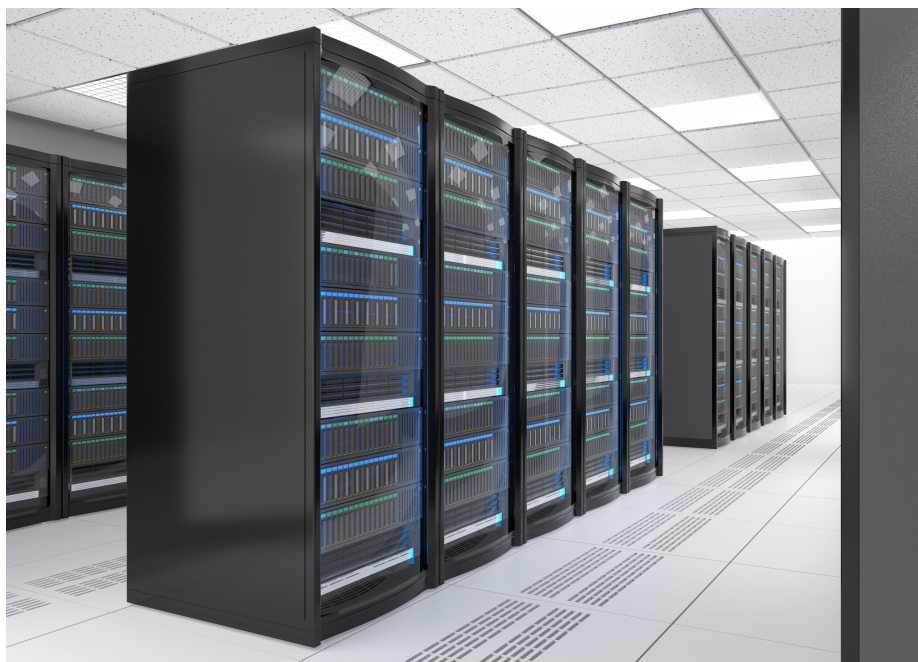
Figure 1.2: Modern server racks where each one is many times more powerful than ENIAC [22]
