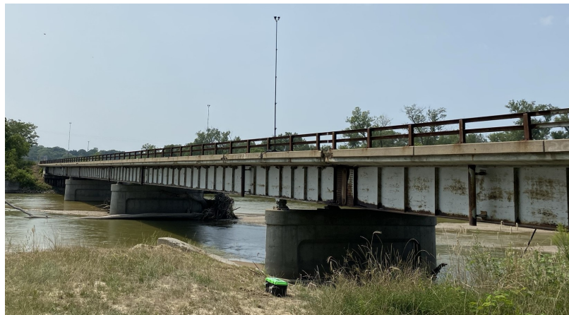
Figure 5.10: East Yutan (EY) bridge.
