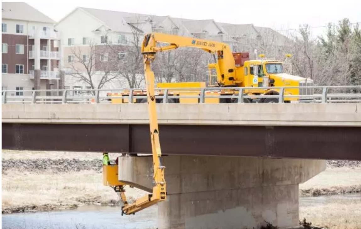
Figure 2.2: Visual inspection of bridge.
